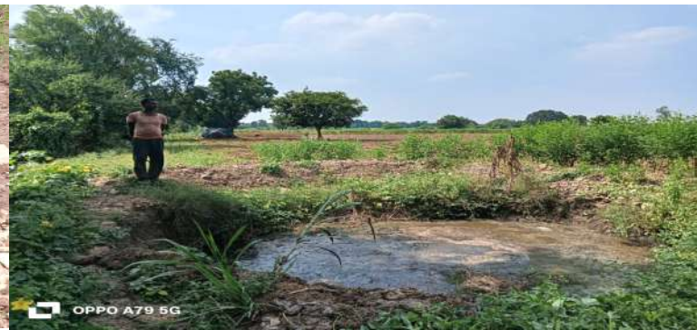
30 Recharge Pits (measuring 15 feet X 15 feet X 10 feet depth) developed with 1.5 million liters water storage
