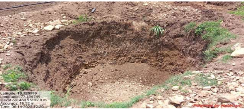
30 Recharge Pits (measuring 15 feet X 15 feet X 10 feet depth) developed with 1.5 million liters water storage
