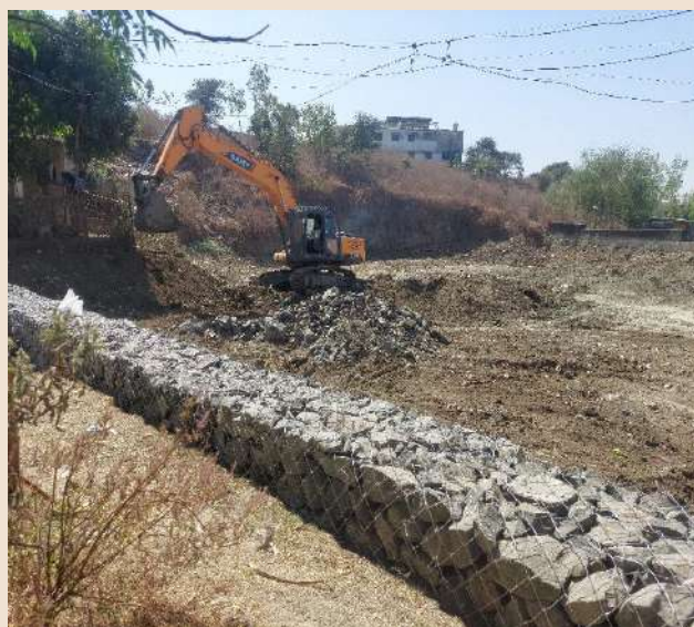
Constructed Staired Gabion
