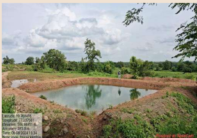
Constructed 10 Farm Ponds, Covered 197 acres of area under irrigation
