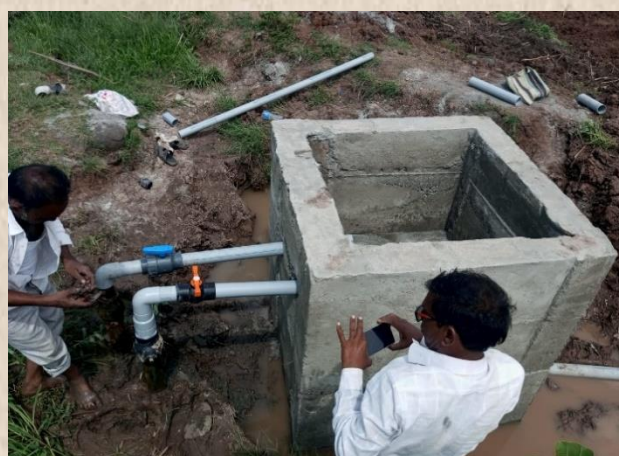
Constructed 2 Diversion-Based Irrigation (PHAD) Units Access for Farmers
